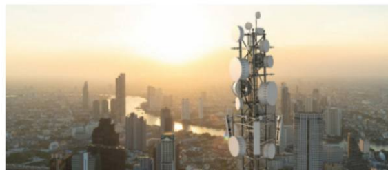
The UK government needs to offer a public/private partnership to catalyse 5G infrastructure deployment.
